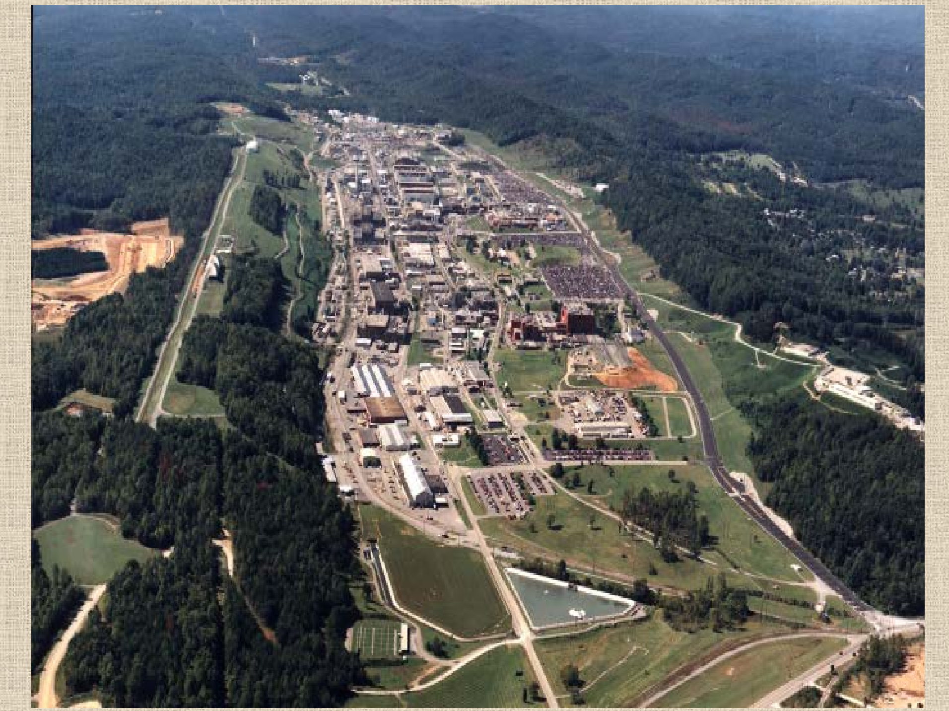
Y-12 National Security Complex, Oak Ridge, Tennessee
